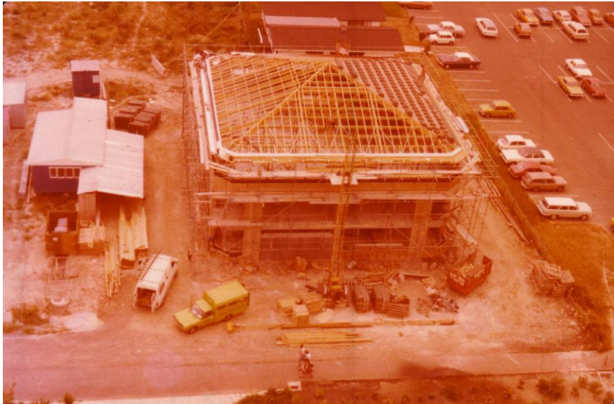
Construction under way
