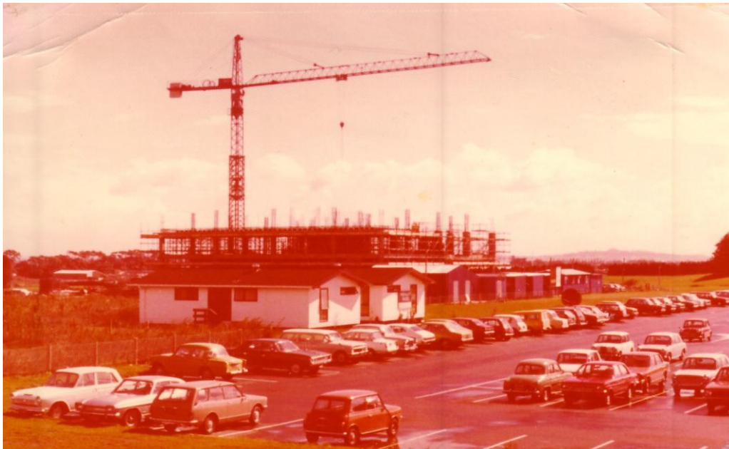
The construction of the permanent building behind the Lockwoods.
